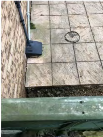
Picture 2 Access Drain in patio at present
